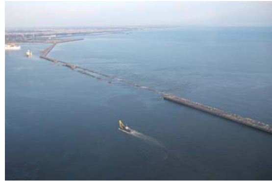
The breakwater was destroyed by the tsunami
